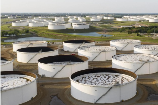
Number of tanks: ~400 Tank diameter: 30-80 m Height: 10-20 m
